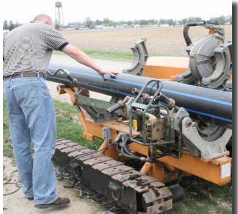
HDPE pipe placed on the fusion machine.
