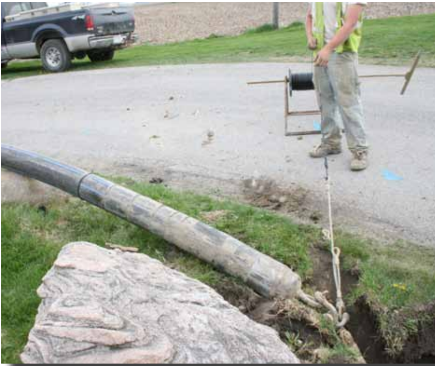
HDPE pipe installed using horizontal directional drilling.
