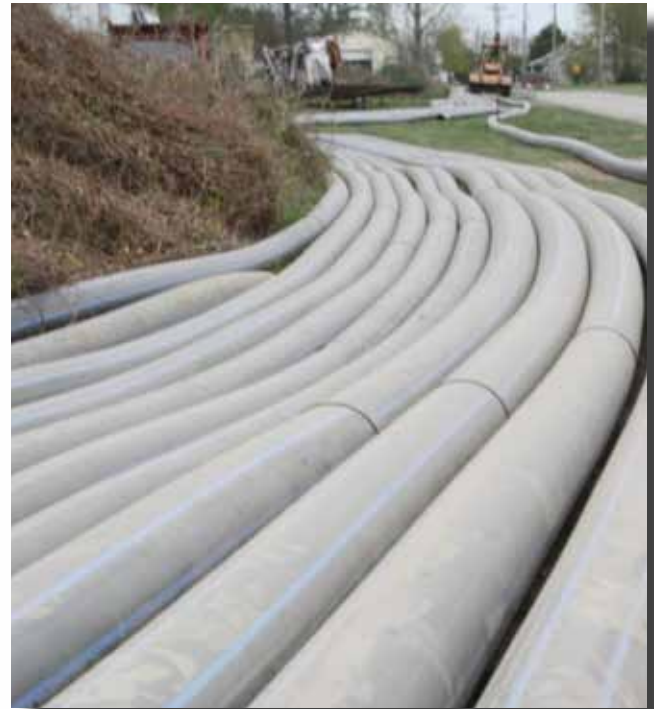
HDPE pipe delivered and laid out for the installation.
