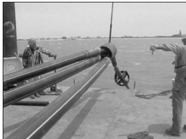
Preparing for Directional Pull.
