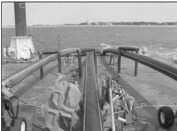
Fusion Machine with Pipe leaving barge.
