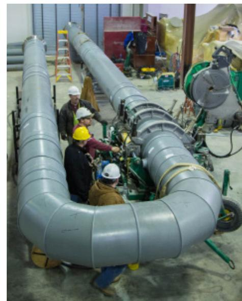
The material is 100% recyclable and environmentally friendly. It also lasts significantly longer than traditional pipe materials because it will not corrode. PP-RCT will outlast the building in which it is installed. "Overall, the idea of thermoplastic pipe for hydronic applications is a sign of the future," said field foreman Scott Rick from Midwestern Mechanical, Inc. in explaining the decision to work with thermoplastics on this project. "It will outlast steel and other types of materials."
